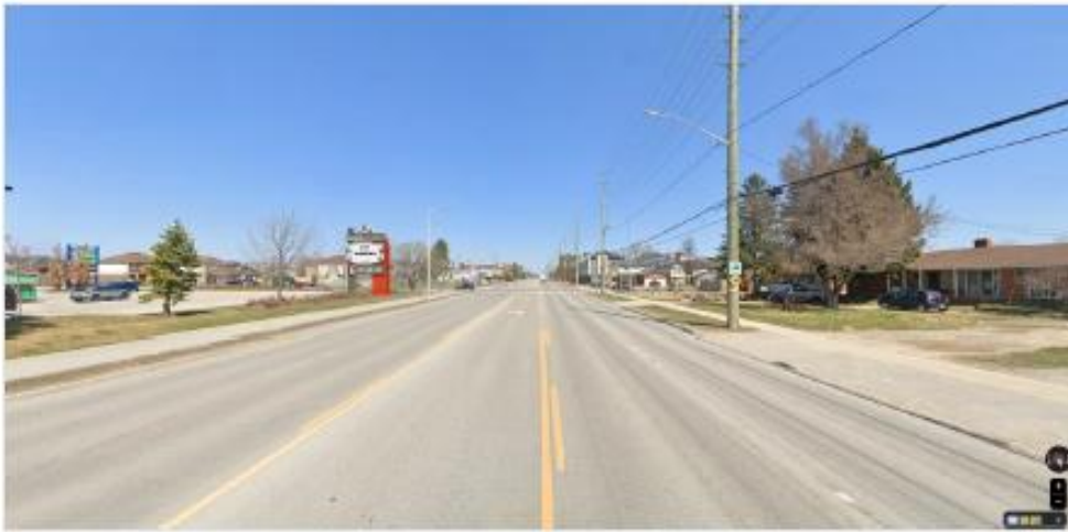
Fig. 1 View looking north along Essa Road
