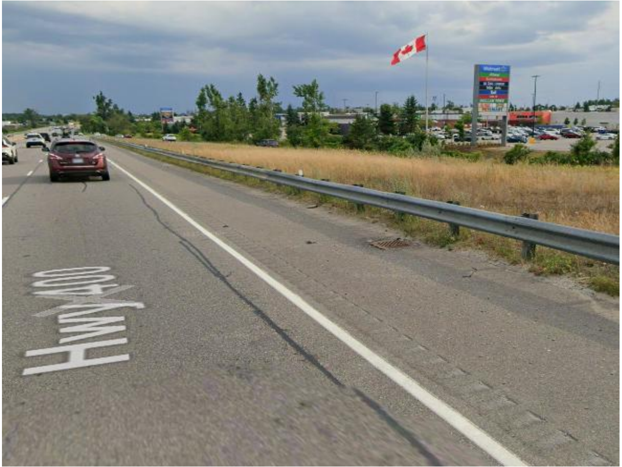
Smart Centre – 35 Mapleview Drive West
